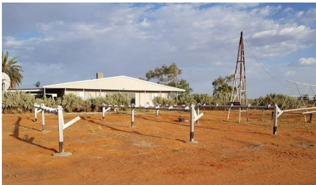
The custom-built 3 seasonal position frames for PV panels takes up an area where a previous solar array stood. A refurbished wind turbine will also feed into the system.
