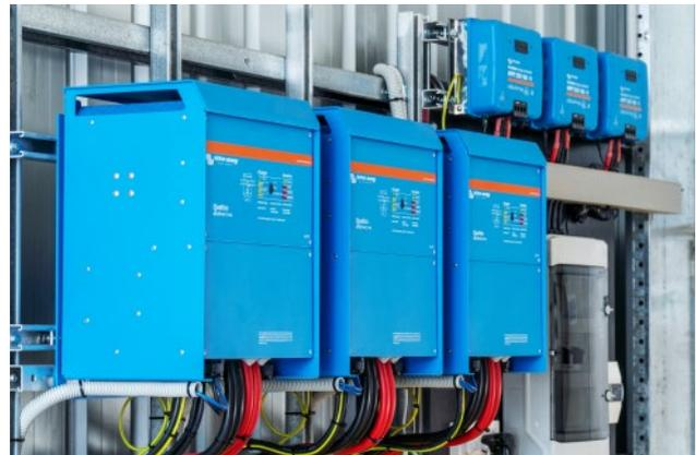
24kVA three-phase consisting 3 x 8000VA Victron Quattro Charger / Inverters
